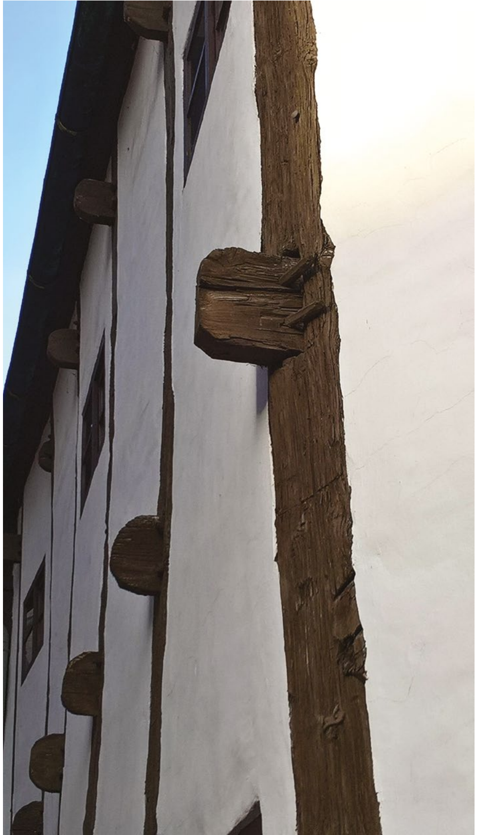
Figure 22. Extended mortise and tennon in the house in Quedlinburg, Wordgasse 3 Source: Elena Perria, 2016.
