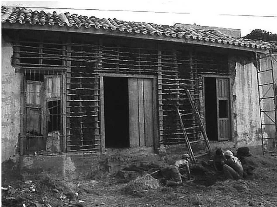
Figure 43. Structure in bahareque technique Source: Revista de la Construcción, 2010.
