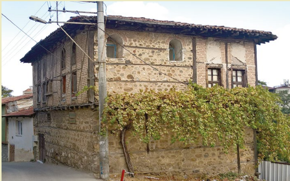
Himş constructional technique on a TAQ technique basement in Mudanya, Turkey Source: Elena Perria, 2017.
