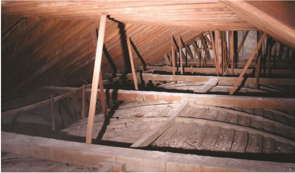
Figure 47. Typical Colonial Roof structure. Cathedral of Santiago de Cuba, Cuba Source: Elena Perria, 2010.
