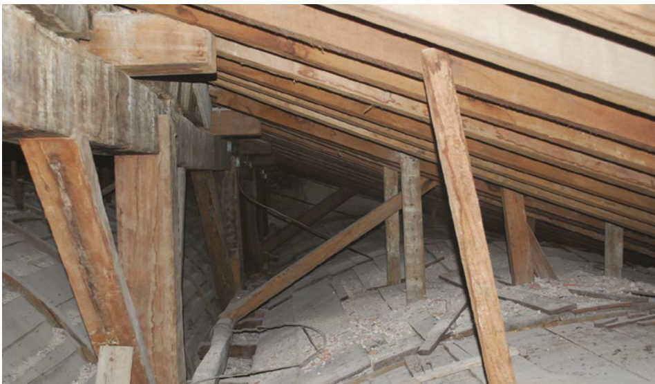
Figure 49. Wooden structure of Santiago de Cuba's Cathedral down into masonry and brick walls Source: Elena Perria, 2010.
