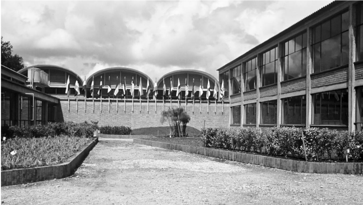
Figura 4. Vista del patio central de la sede del CINVA a los pocos meses de su inauguración. Fuente: Currie, Leonard J. (Leonard James), 1913-1996 (Photographer), "CINVA (Inter-American Housing and Planning Center), Bogotá, Southwest Virginia Digital Archive, accessed June 9, 2022, https://di.lib.vt.edu/items/show/676 .
