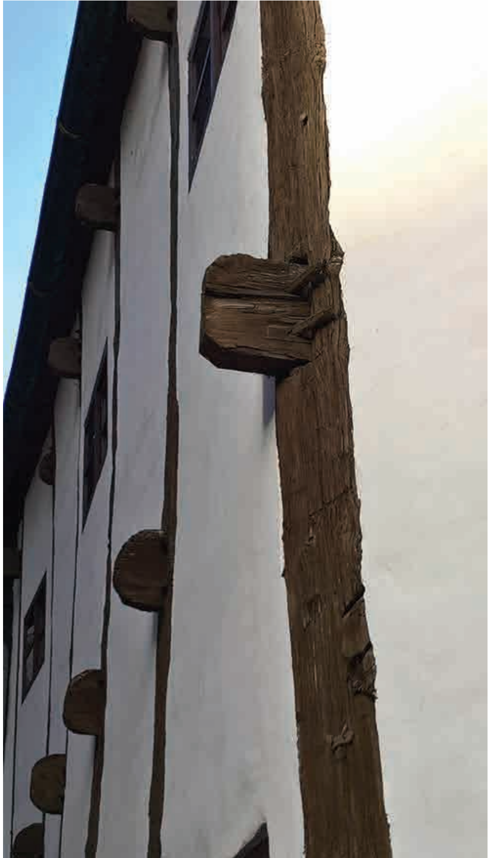
Figure 22. Extended mortise and tennon in the house in Quedlinburg, Wordgasse 3 Source: Elena Perria, 2016.
