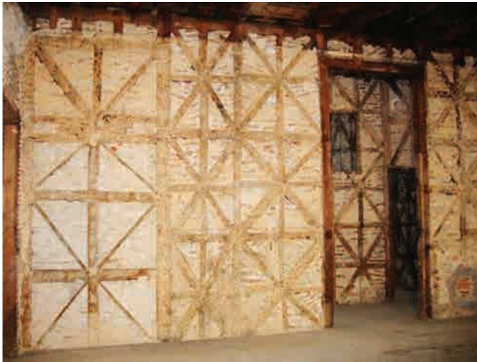
Figure 11. Gaiola Pombalina Source: Monumenta, Poletti, 2013.
