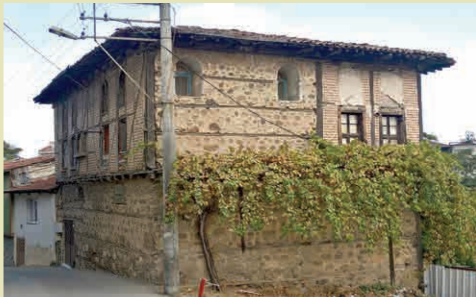
Hımsı constructional technique on a TAQ technique basement in Mudanya, Turkey Source: Elena Perria, 2017.
