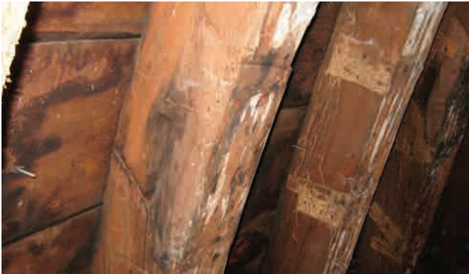
Figure 48. Jupiter joint or Splayed undersquinted and tabled scarf joint with key of the wooden dome of Santiago de Cuba's Cathedral, Cuba Source: Roncoli, 2013.
