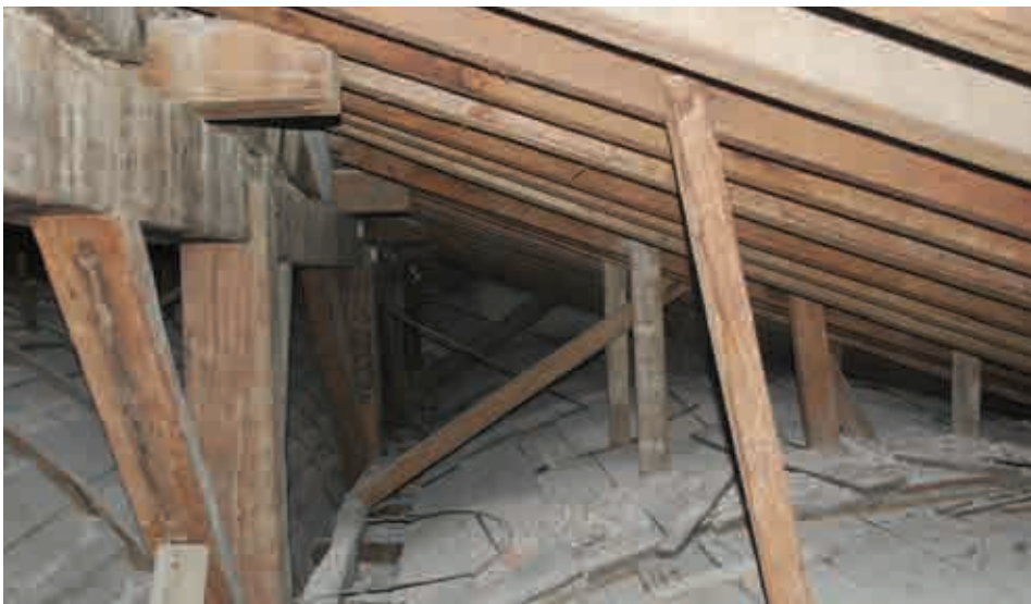
Figure 49. Wooden structure of Santiago de Cuba's Cathedral down into masonry and brick walls Source: Elena Perria, 2010.
