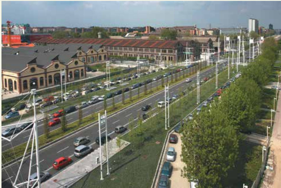
Figure 3. The “Central Backbone”: the new inner boulevard built after the lowering of the railway tracks. It is one of the main urban transformation that started with the approval of the General Plan in 1995. Photo by M. D’Ottavio
