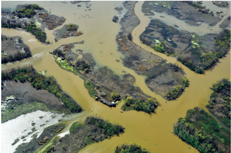
Figure 8. Pipeline structure in remote section of wetland Source: image by author.
